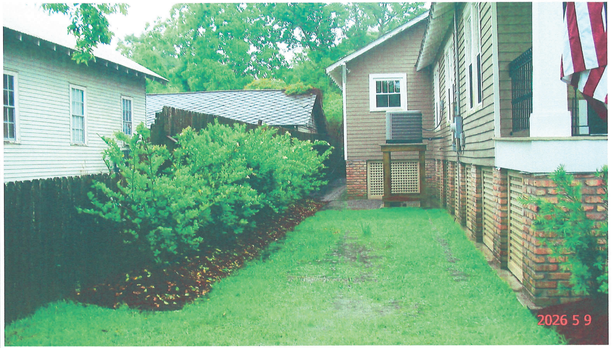
5/9/2026 1:37 PM Total Site Inundation (wide view)
