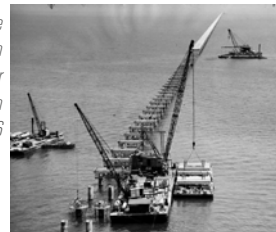
Lake Ponchartrain Causeway under construction in June 1956
