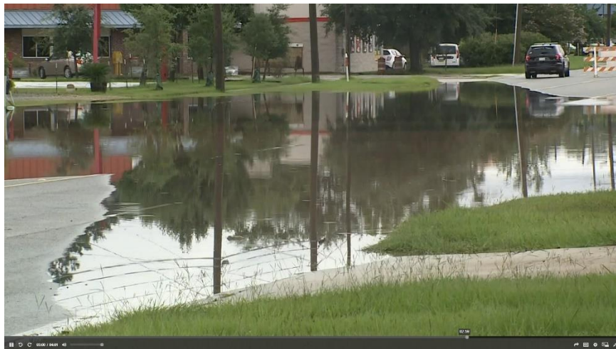
Figure 3-6: Flooding at Florida Street
