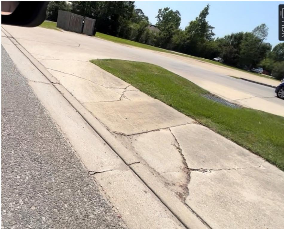
**Figure 4-36: Giron Street Cracked Sidewalk Panels**
