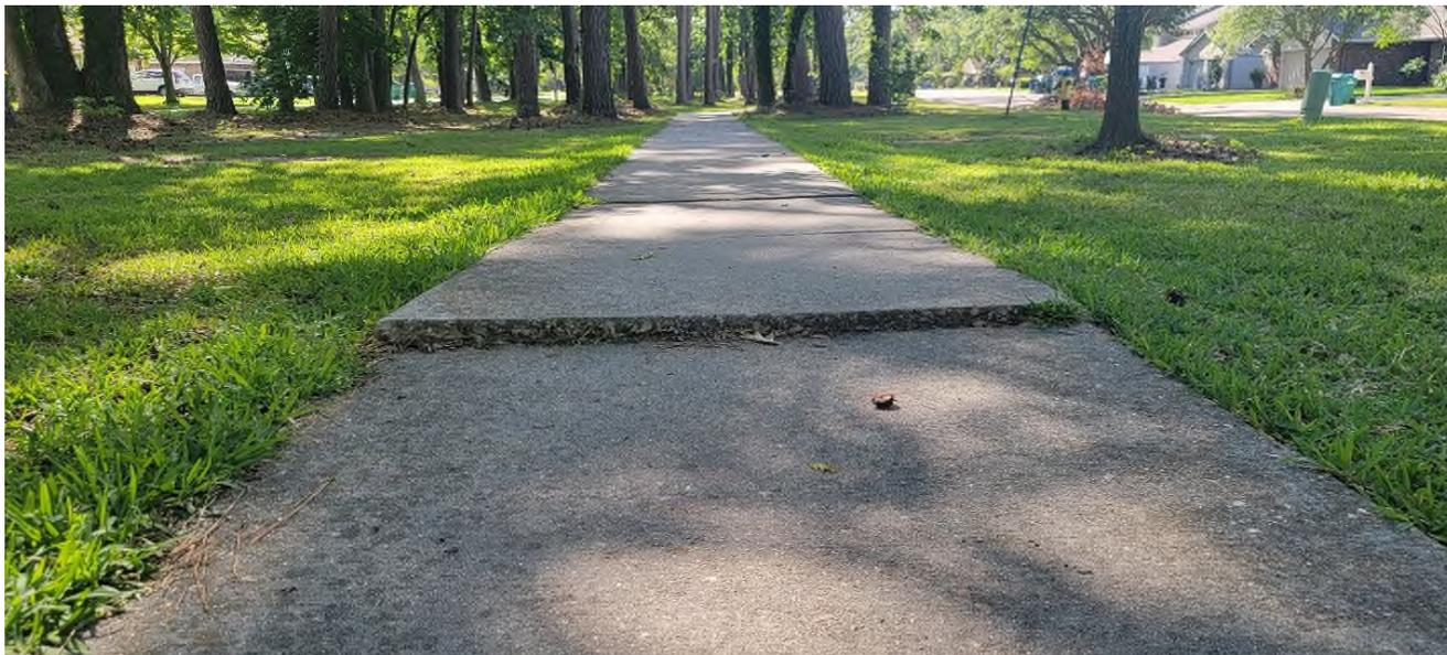
**Figure 4-19: Concrete Sidewalk Slab Elevation Differential (Monroe Street)**
