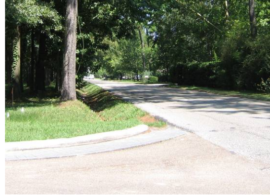
Drainage swales preclude the installation of sidewalks or bike lanes along some streets.
