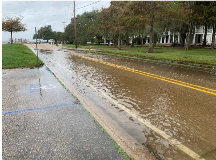
Flooding on Lakeshore Dr. despite otherwise dry streets and no active storm events; high water levels in Lake Pontchartrain can push water back through the drainage system.
