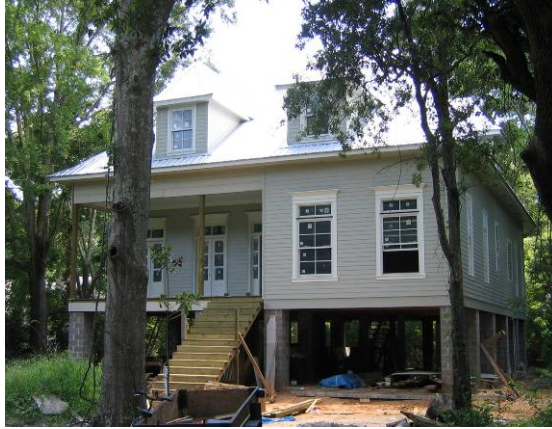
FEMA recommends elevating structures by 12 feet or more in some parts of Mandeville.
