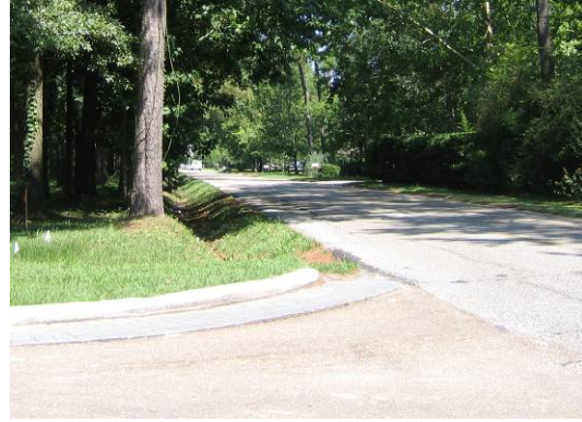
Drainage swales preclude the installation of sidewalks or bike lanes along some streets.
