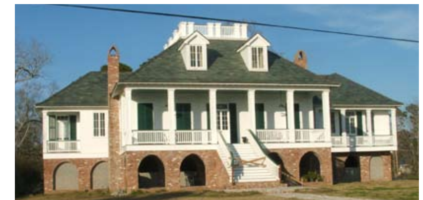
5 Major Elements 4 Minor: Side Porch, 2 Dormers, Widows Walk
