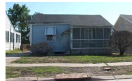
Entry facing driveway
