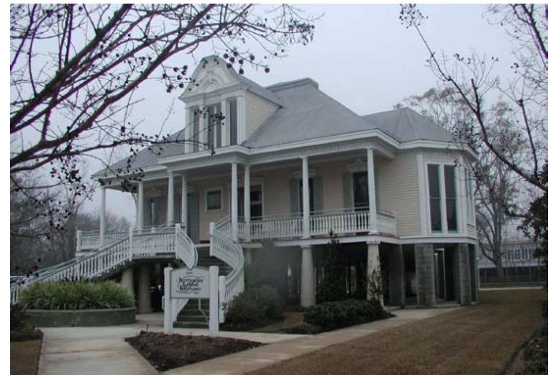
Transition using a Porch, Stairs, Railings, and Landscaping.
