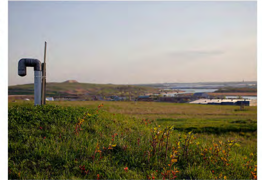
Landfill Cap Freshkills Park, Staten Island, NY
