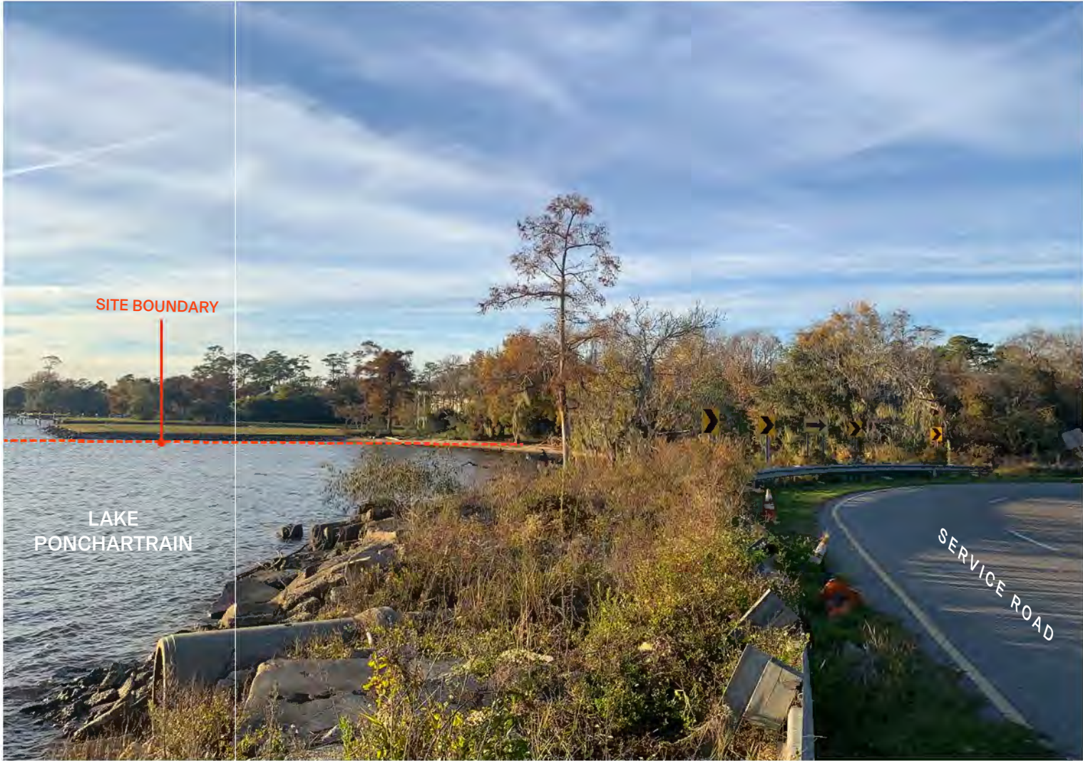
Existing site from Causeway Service Road at Toll Plaza
