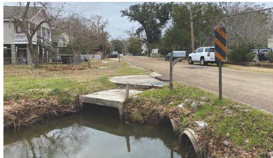
Ravine aux Coquilles channelized underneath Carroll Street
