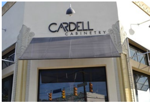
Figure 10.3.7: Externally Illuminated Sign Example.
