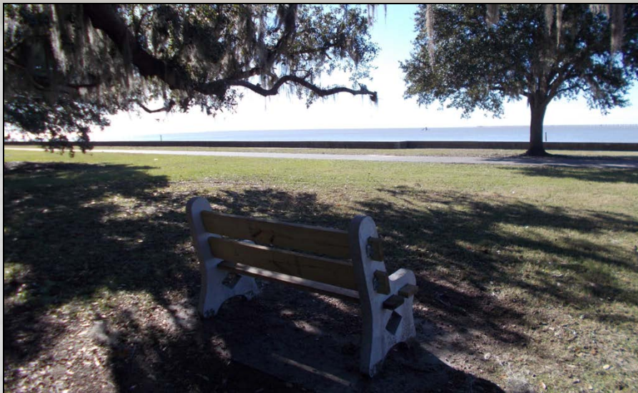
View of Existing Seawall, El. 5.3
