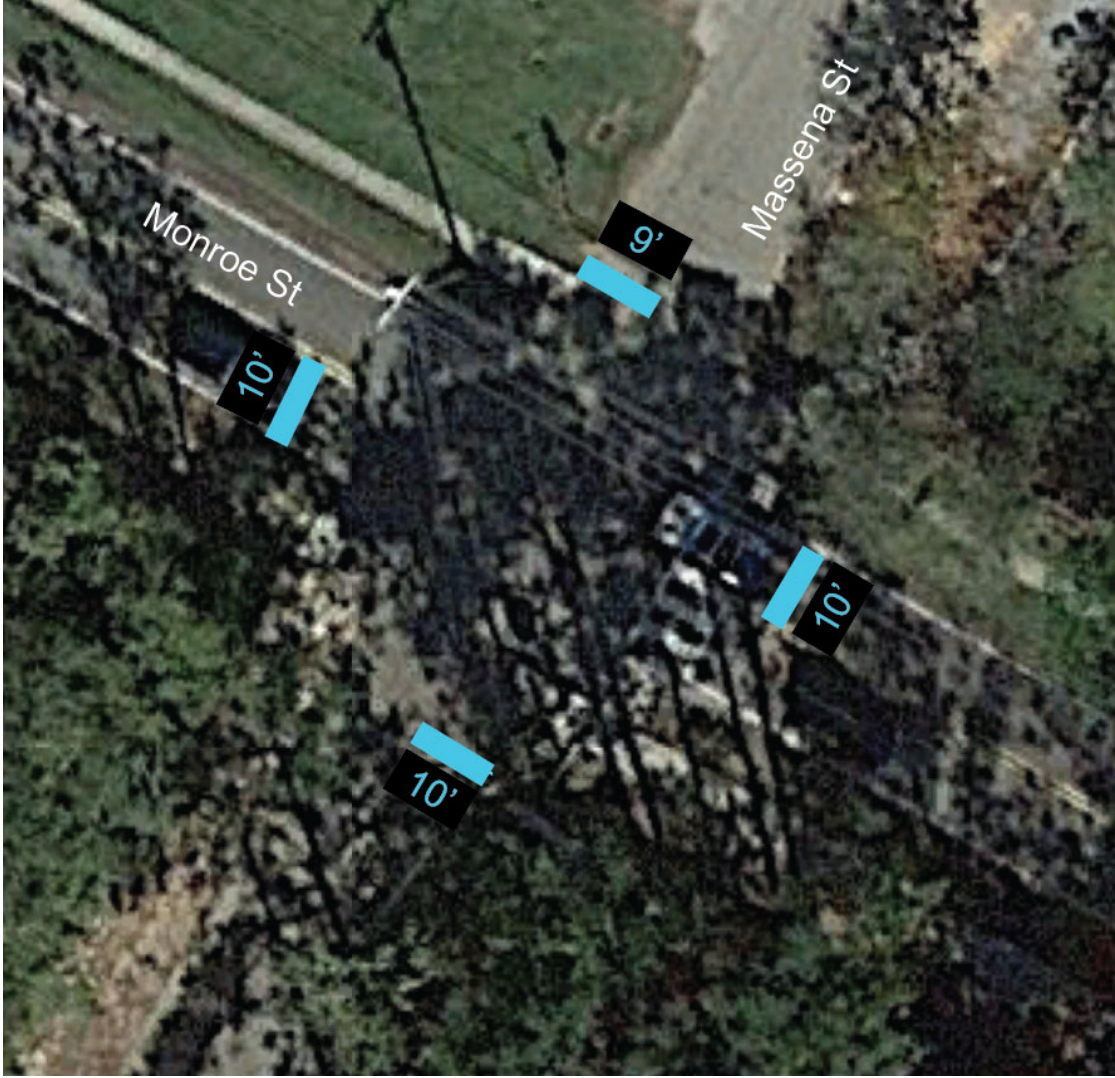
Photo 5 – Massena St at Monroe St
