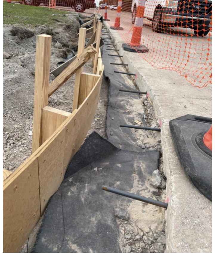
Without #6 smooth dowels, Lakeshore Drive (North). With #6 Smooth Dowels, Lakeshore Drive (South)
