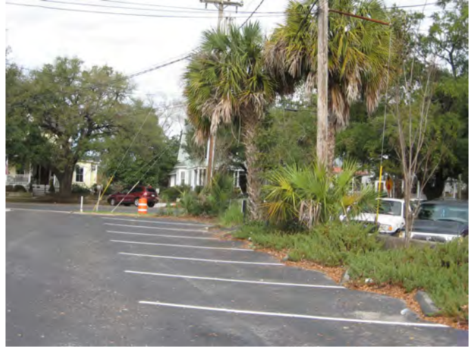
Landscaping introduced into this parking lot would help define the parking spaces and reduce water runoff.
