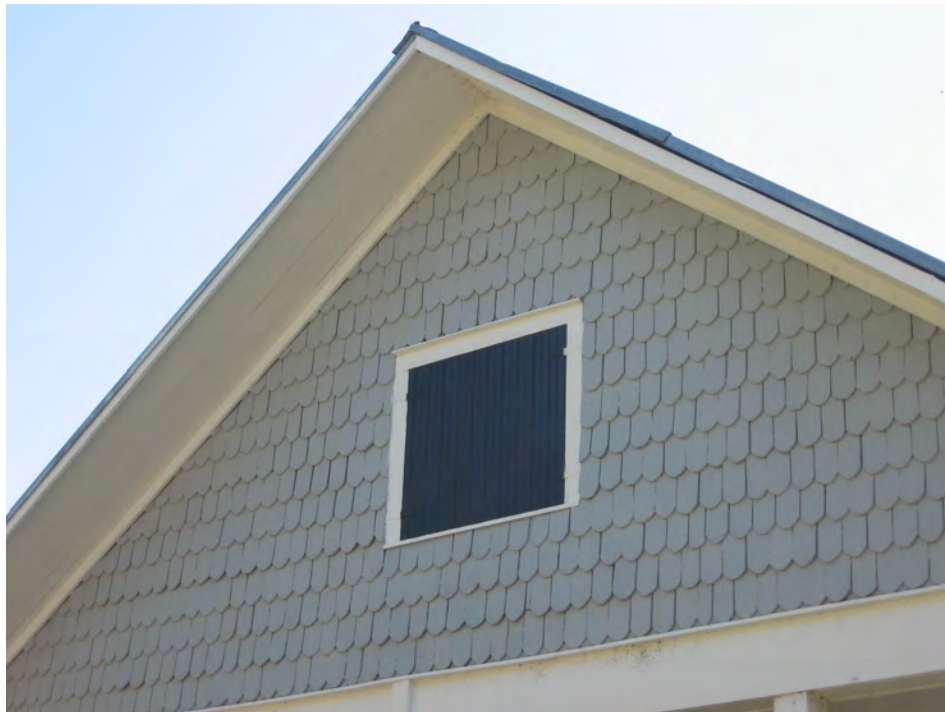
Wood shingles were widely used in Mandeville as exterior siding materials for upper floors and gables (413 Girod Street).
