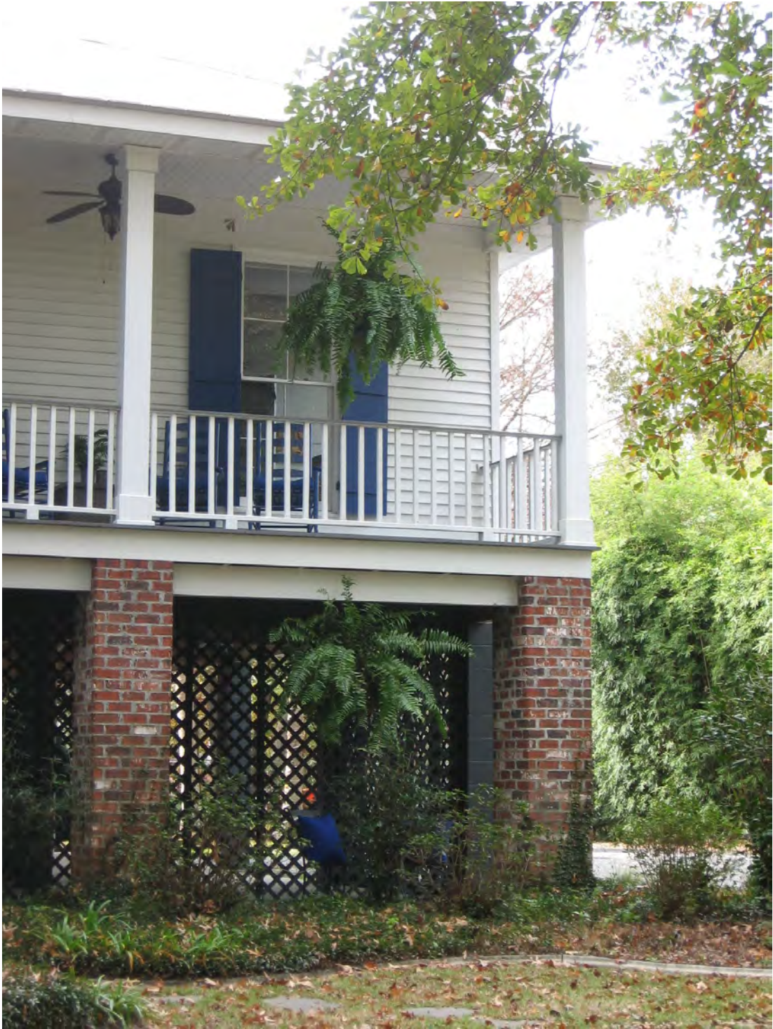
The dwelling at 2610 Jefferson Street illustrates appropriate alignment of the porch columns with the foundation piers below as well as recessed lattice panels and screening.
