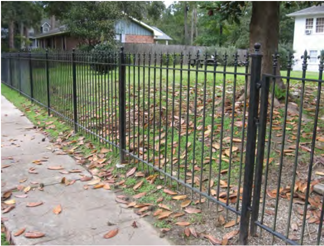
At left is an example of an appropriate modern fence close to the street that is taller than three feet but allows for visibility through the fence for driving safety at 263 East Street.
