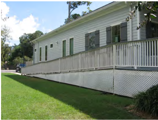
For residential properties converted to commercial or offices use, ramps should be sited on rear or side elevations such as this ramp at 419 Girod Street.
