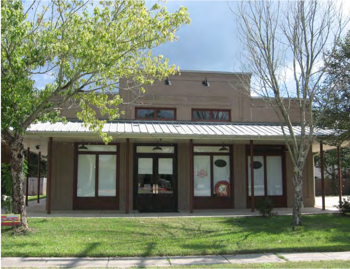
The new construction at 821 Marigny Avenue was designed with a stepped parapet wall and traditional storefront appropriate for the district.
