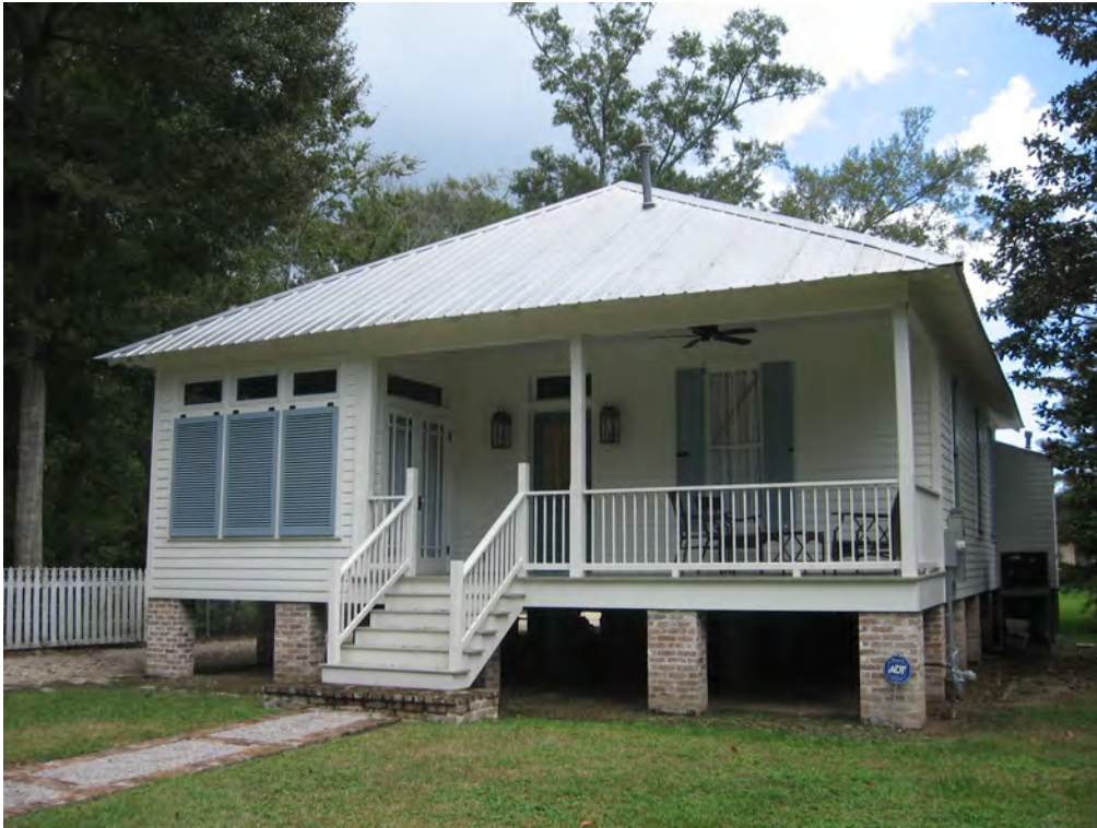
The dwelling at 551 Carroll Street is on a brick pier foundation. Brick pier foundations can be both open or enclosed with lattice panels.
