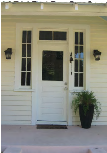
Entrances with original sidelights and transoms should be preserved (left, 1932 Jefferson Street). The wood-panel door at 317 Girod Street features a single-light with a multi-light stained-glass border (center). An appropriate screen door for a porch entrance is at 219 Lafitte Street (right).
