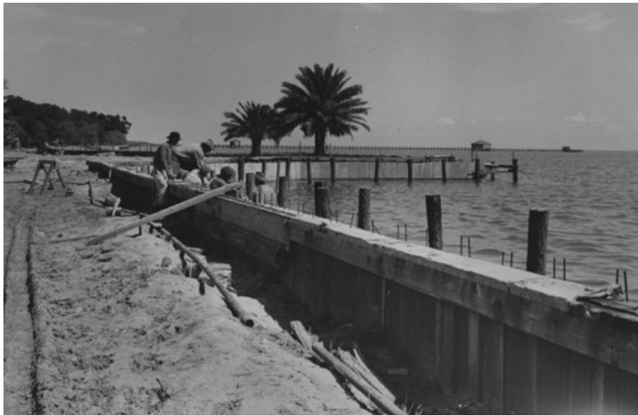
Construction of the sea wall in 1937.
