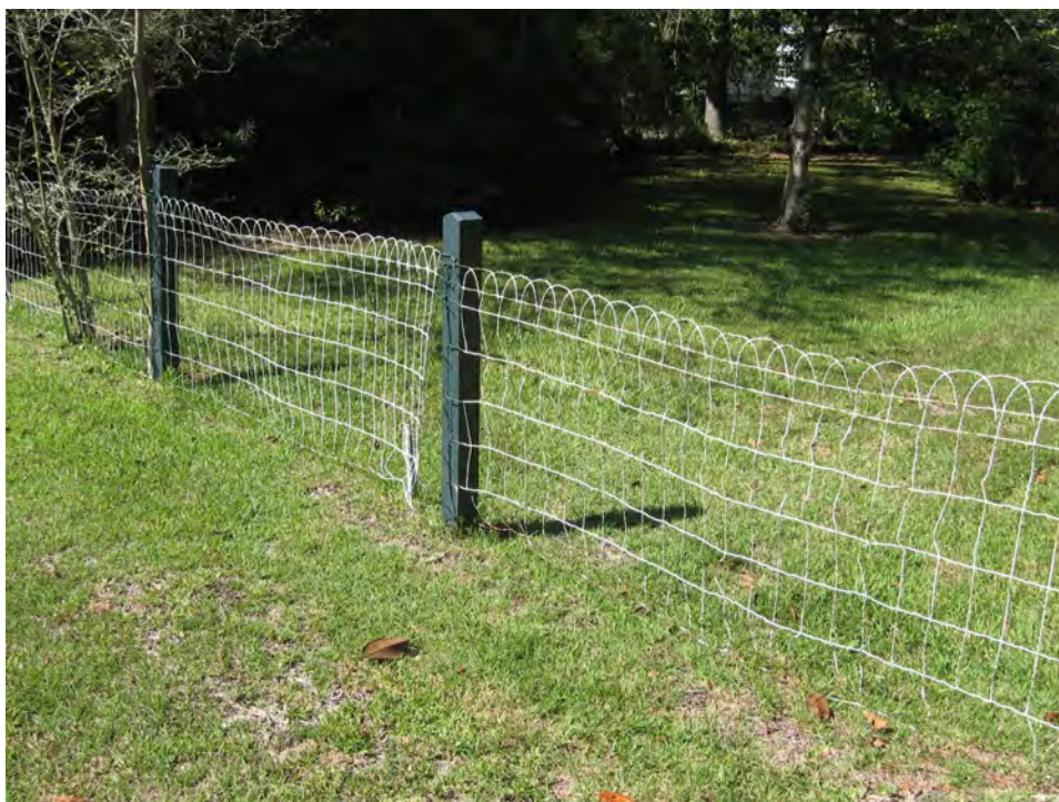
Several dwellings retain early twentieth century wire fences (504 Marigny Avenue).
