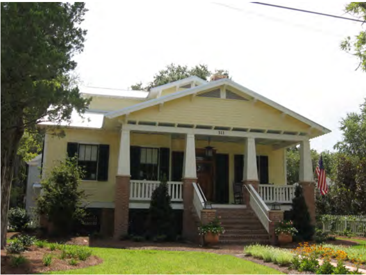
Further from the lake front infill construction can be at-grade or a few feet above grade. At left, a Bungalow infill dwelling at 311 Lamarque blends with historic dwellings on the street. The house at 650 Lamarque Street (right) is based on the North Shore type with a lateral rear wing.
