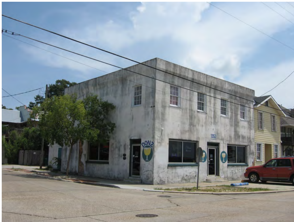
Stucco was applied as a protective coating over the brick on this ca. 1850 commercial building at 1951 Lakeshore Drive.
