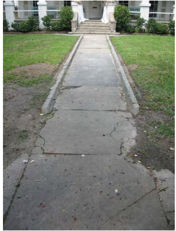
Original concrete walkway at 402 Lafitte Street.
