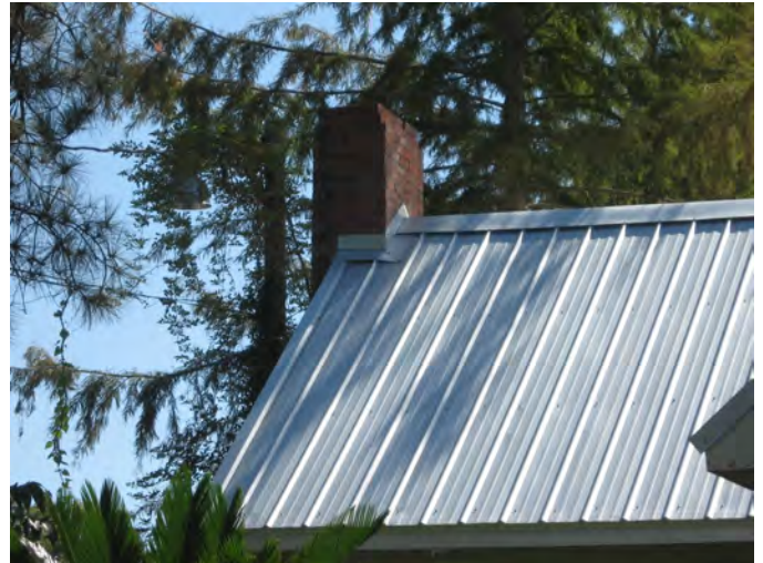
These dwellings in the historic district have replacement metal roofs of appropriately sized crimping and spacing in traditional metal roof designs 501 Marigny Avenue (left), 321 Girod Street (right).
