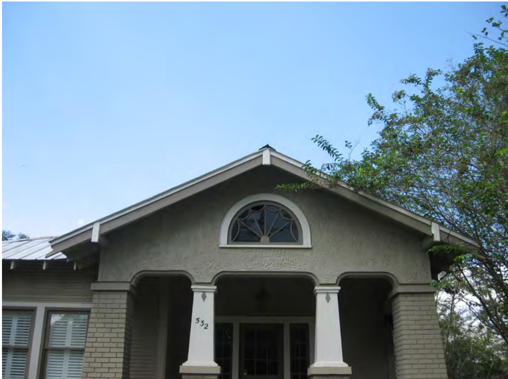
The Bungalow dwelling at 532 Girod Street has original stucco in the gable field which is an important part of its character.
