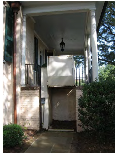
This chair lift design provides access from a dedicated parking space, is screened by landscaping and required only a small section of the porch to be removed.
