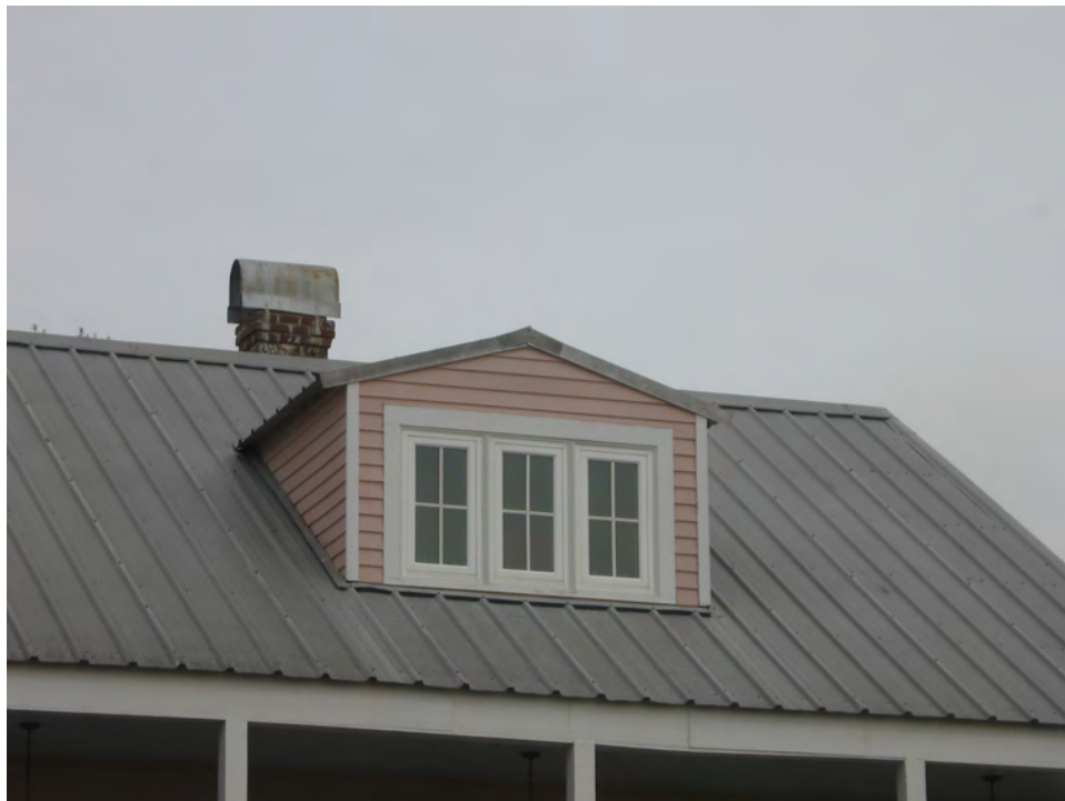
Example of an appropriate corrugated metal roof (1725 Lakeshore Drive).
