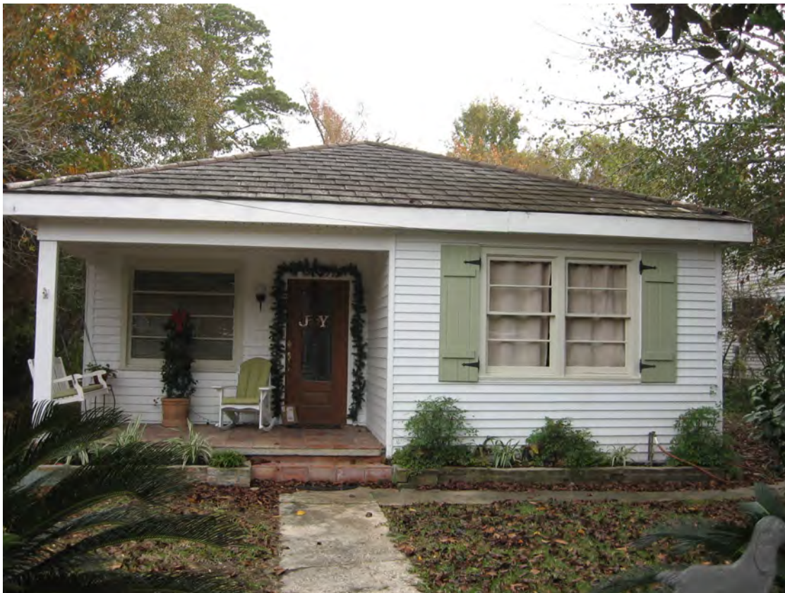
During the 1950s a number of Minimal Traditional style dwellings were built in the historic district. These were typically designed with restrained detailing and one-story in height (547 Marigny Avenue).
