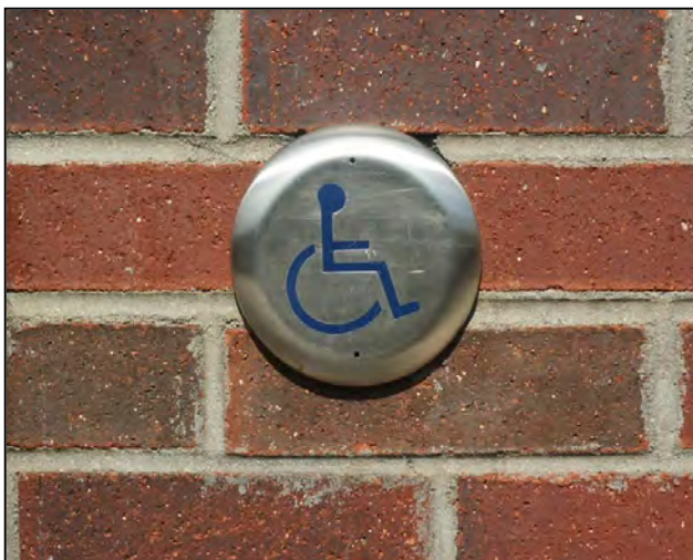
Original doors on commercial buildings can generally be retrofitted with push plates (left) which activate door openers (right) to allow wheelchair access.
