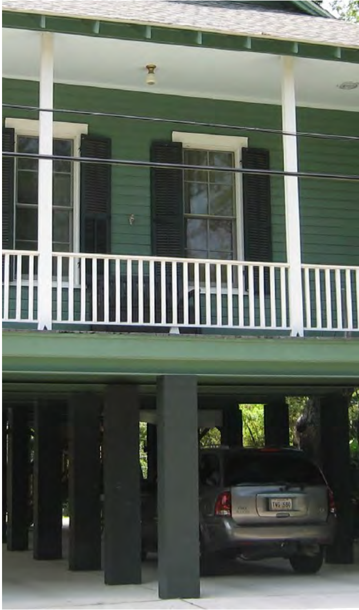
NO: The porch columns and foundation piers on these structures do not align.
