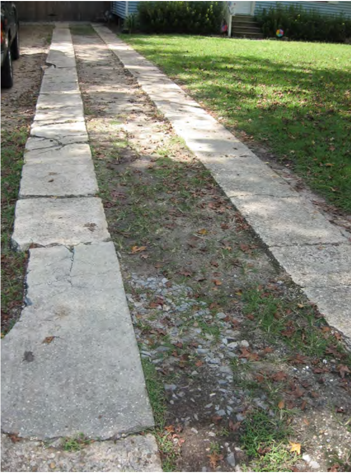
Historic concrete ribbon driveway at 306 Marigny Avenue.
