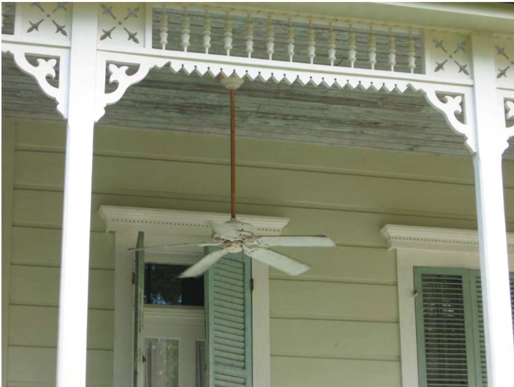
Mandeville's dwellings from the nineteenth and early twentieth centuries have distinctive wooden valances like the lattice design at 319 Lafitte Street (above) and the milled and jigsawed wood details at 330 Marigny Avenue (below).
