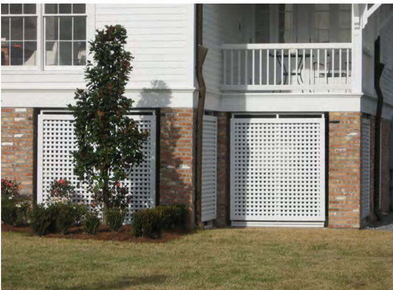
YES: These breakaway lattice panels are appropriately placed between the brick piers.
