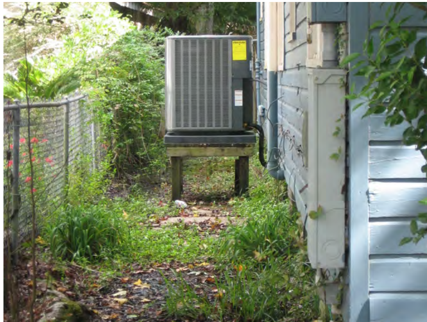
HVAC units should be sited at rear or side yards as at 276 East Street (above) and 335 Marigny Avenue (below). Both units are elevated above grade to avoid flooding.
