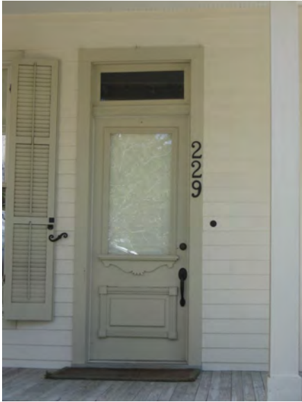
Many of the oldest dwellings in the historic district display original single-light glass wood doors with detailed designs and transoms such as at 229 Lafitte Street (left), paired multi-light glass and wood doors such as at 2017 Jefferson Street (center), and entrances with decorative surrounds such as this Classical entrance at 149 Coffee Street (right).
