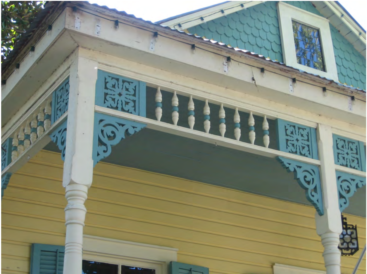
Bright paint colors highlight the detailed wood trim of 19th century Victorian-era dwellings such as the dwelling at 317 Girod Street.
