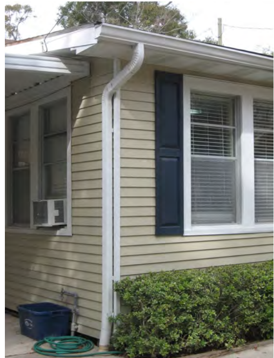
Example of appropriate gutters and downspouts at 326 Marigny Avenue (left) and 316 Girod Street (right).
