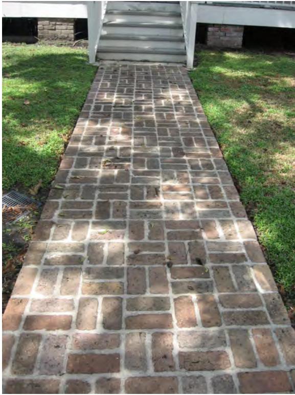
The installation of brick pavers laid in traditional patterns is appropriate for new walkways (212 Lafitte Street).
