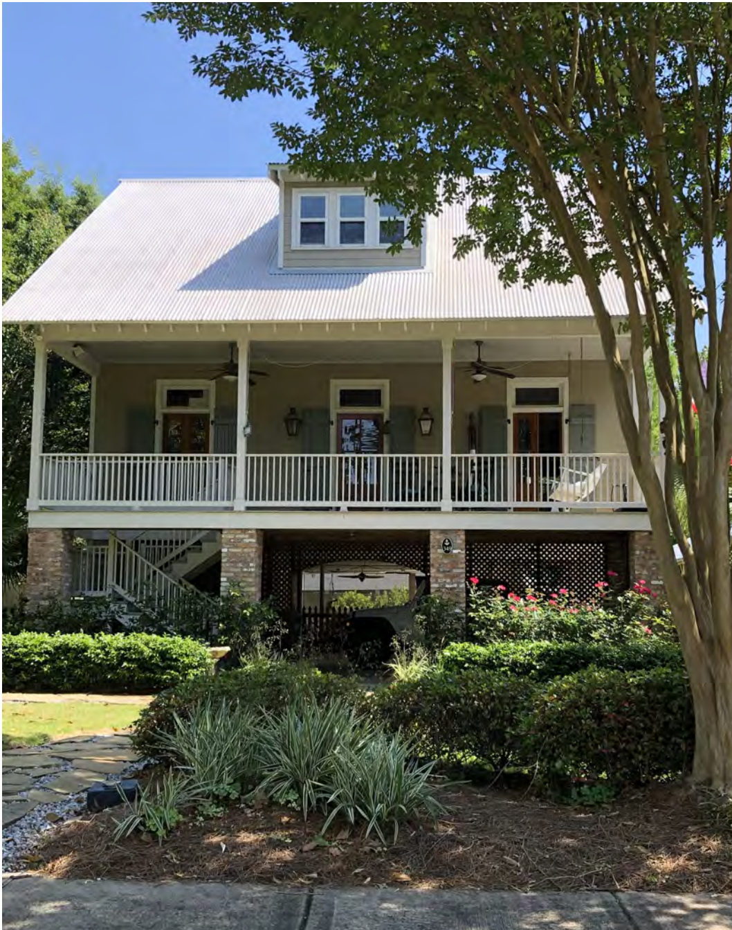
This elevated new dwelling has appropriately sized porch columns with bases and capitals, an interior staircase, full-width porch and dark screening placed behind the fascia board (349 West Street).
