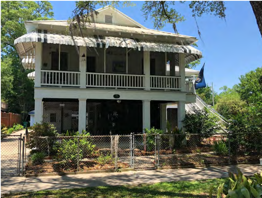
The dwelling at 138 Marigny Avenue has lattice panels which are placed in line with the front wall of the house and behind the porch.
