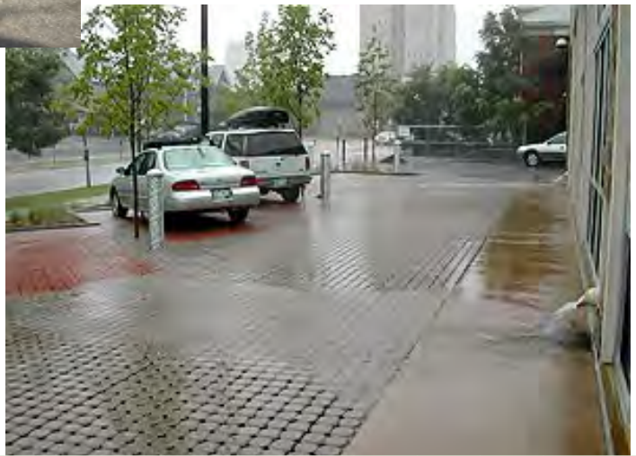
When installing new parking lots or repaving existing ones, the use of permeable paving materials is encouraged to permit water absorption and help limit ponding on surfaces.
