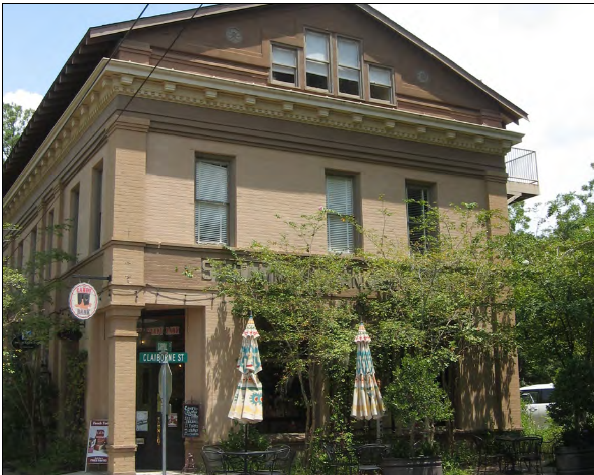
The St. Tammany Bank built in 1907 at 201 Carroll Street is the most traditional early twentieth century commercial building in Mandeville.
