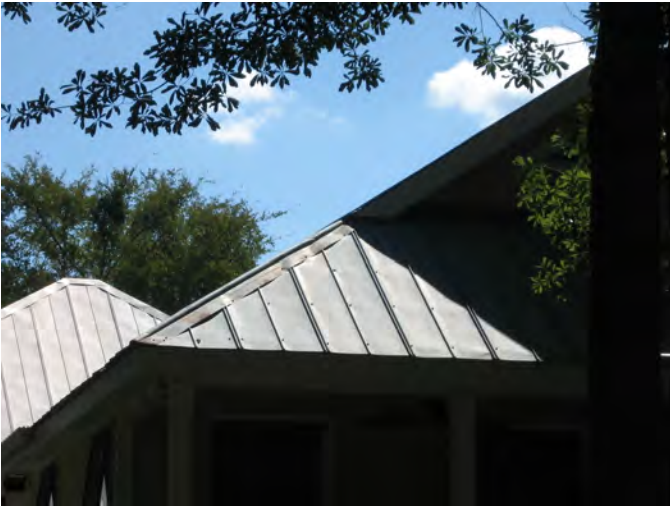
These dwellings in the historic district have replacement metal roofs of appropriately sized crimping and spacing in traditional metal roof designs 501 Marigny Avenue (left), 321 Girod Street (right).
