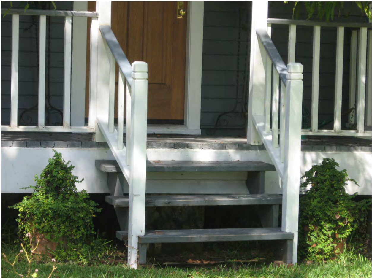
This wood stair is an appropriate design with its square newel posts and balusters (604 Marigny Avenue).
