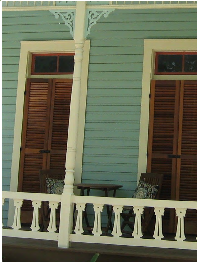
Full-height louvered shutters at 211 Girod Street.
