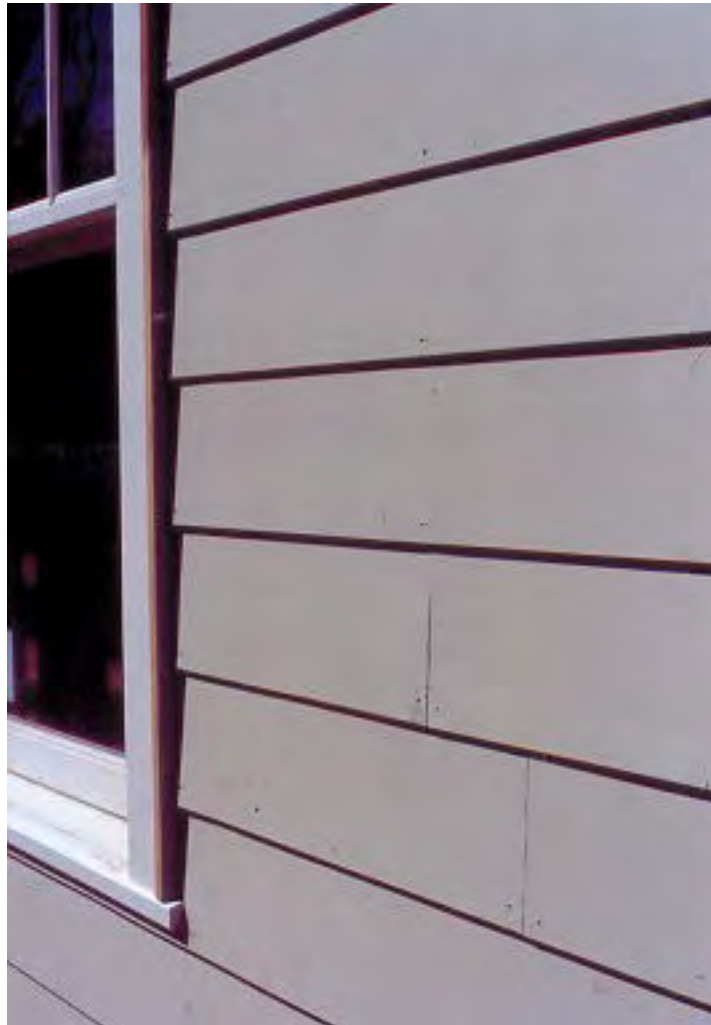
Cementitious siding is an alternative material that may be appropriate in some circumstances.
