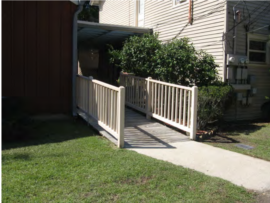
Appropriate ADA ramp at the rear of 347 Girod Street.
