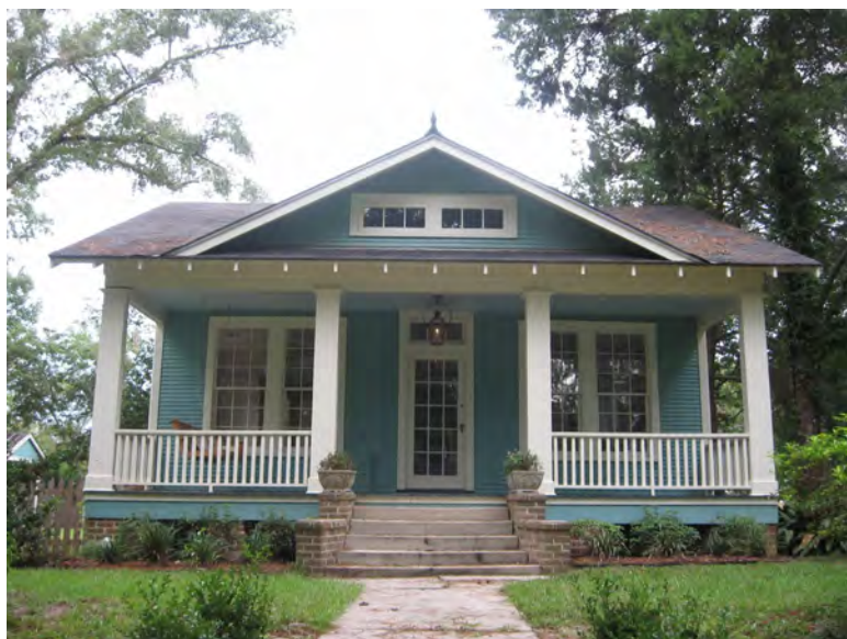
Porches are important character defining features and should not be enclosed on primary facades with glass or other materials (276 East Street).
