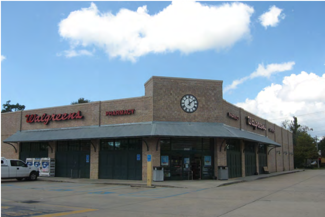
This drug store on Florida Street was designed with a brick exterior, stepped roofline, bracketed awning and traditional storefront for compatibility with the district.
