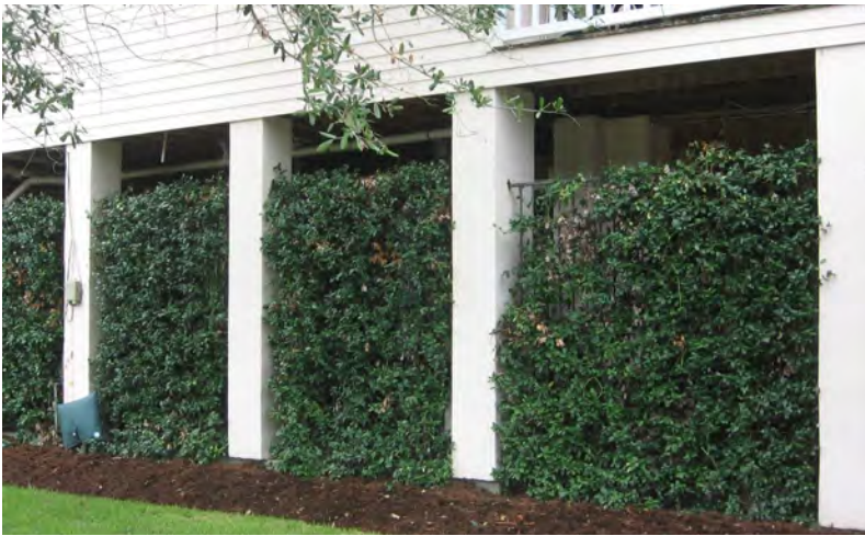
YES: Landscaping between the piers of an elevated foundation creates a screening effect.
