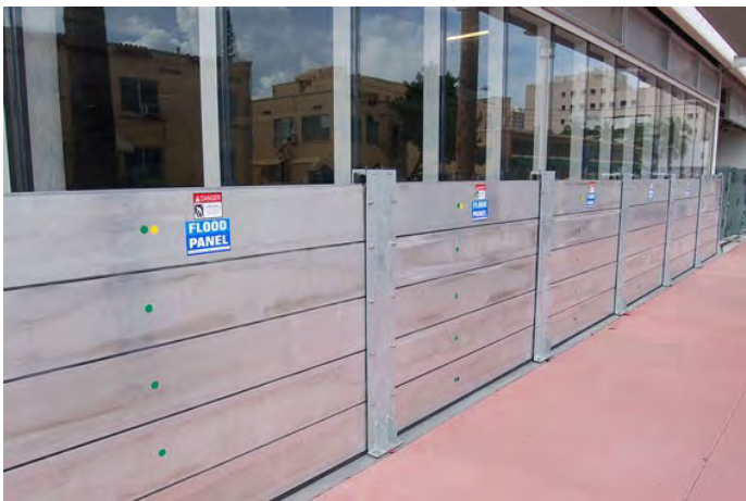
Temporary flood panels are now widely available for historic commercial buildings. When high water events are anticipated these can be erected to minimize flood damage.
